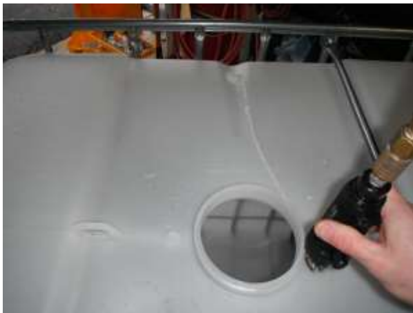
Mark 4" from inside rail centered from front to back...
